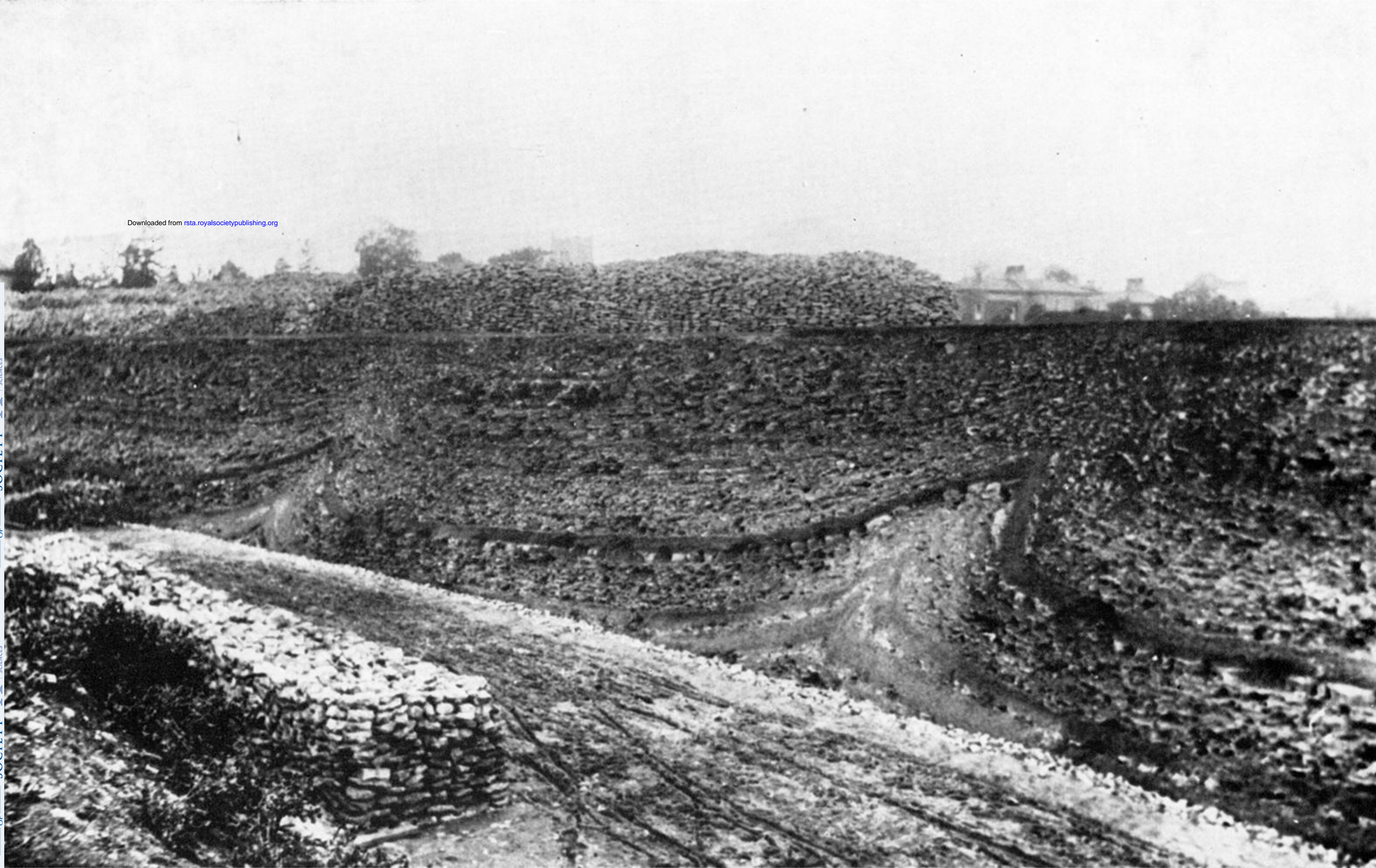
FIGURE 17. Valley-bulge structure in Lias clay near Keynsham. Undisturbed gravels of the overlying no. 2 Terrace had been removed by excavation before the photograph was taken (photo by J. W. Tutcher ca. 1922). The section is 6\frac{1}{2} m high.
